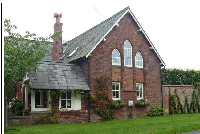
The Old School Porch and Windows
