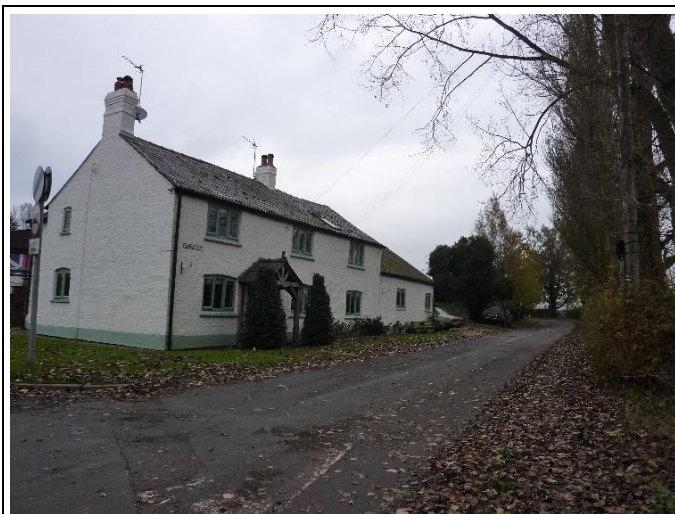
View South down School Lane from Chelford Road with Smithy Cottage
