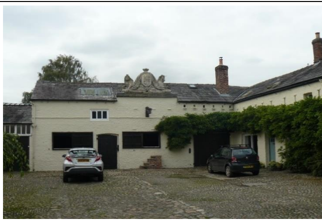
Stable Block, Ollerton Lodge (Converted Stable Cottage to Right)
