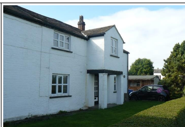
North End (Part of Beeches Farm)
