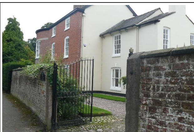
Three Storey Ollerton Lodge
