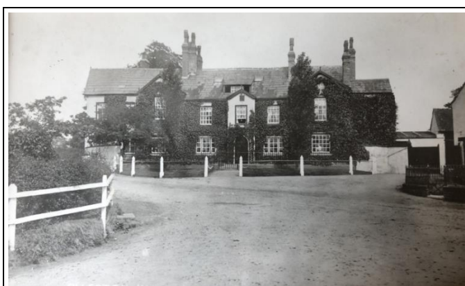
Ollerton Hall Front Elevation ca. 1914
