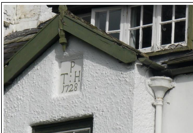
Original Casement Windows, Ollerton Hall
