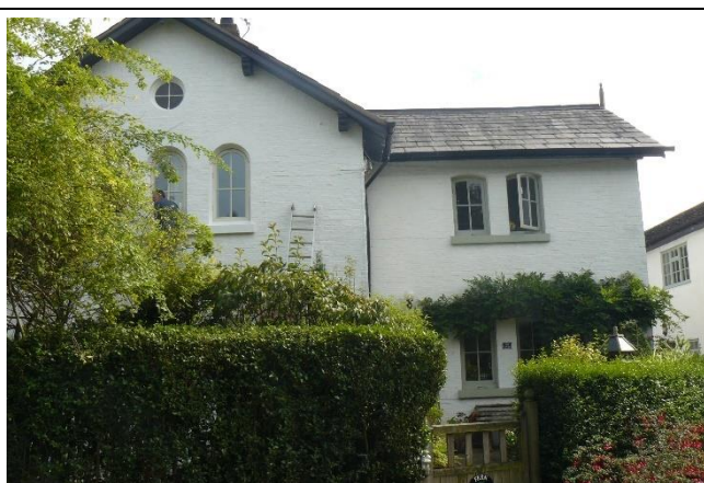
New Windows in Original Openings
